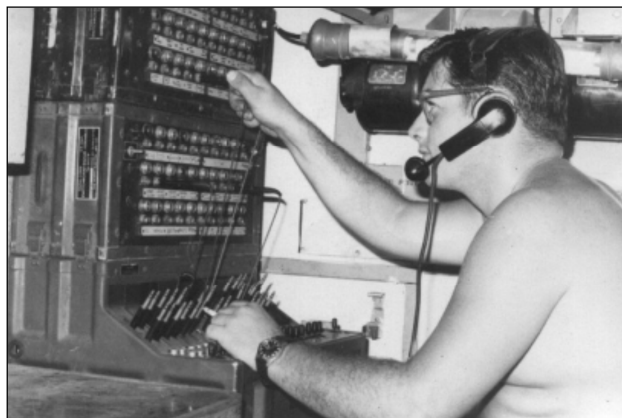
Photo 4.9 (left) - Signalman Reginald Dando operating Ebony Switchboard AN/MTC-7 Shelter (1966)
