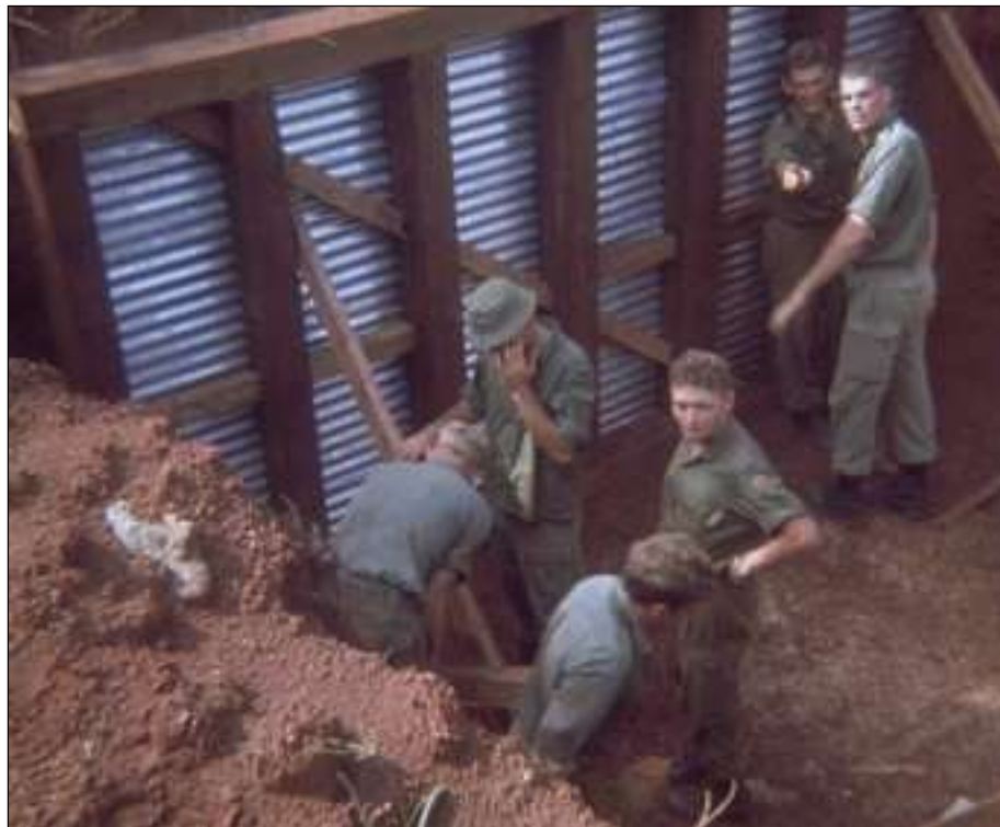
Photo 7.5 - 104 Signal Squadron members digging the COMMCON bunker (Late 1968).
