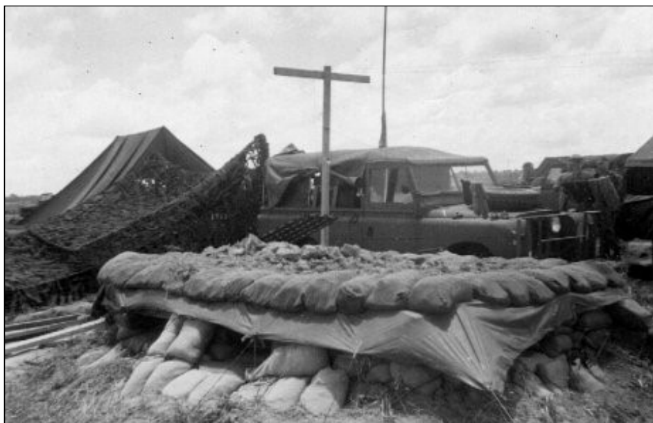
Photo 2.5 - AN/TRC-75 Vehicle and main 709 Bunker at Bien Hoa (July 1965).
